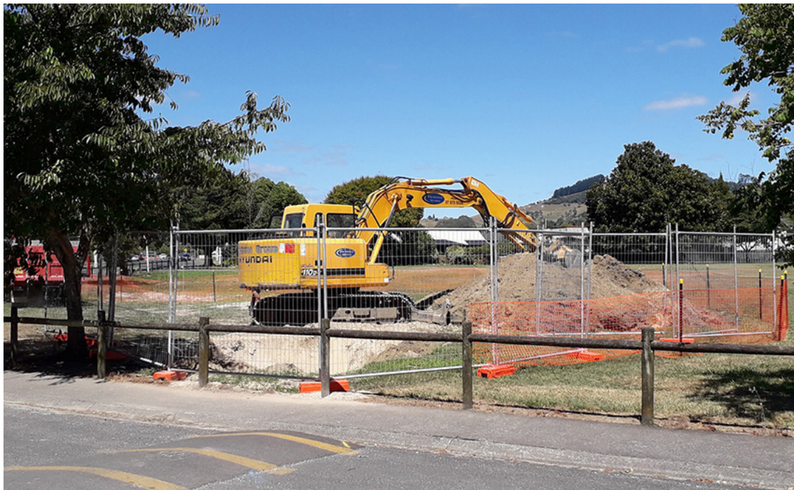
EARTHWORKS FOR SEWER MAIN REPLACEMENT AT TE KUITI DOMAIN
