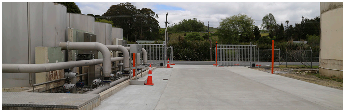
NEW ENTRANCE AT TE KUITI WATER TREATMENT PLANT
